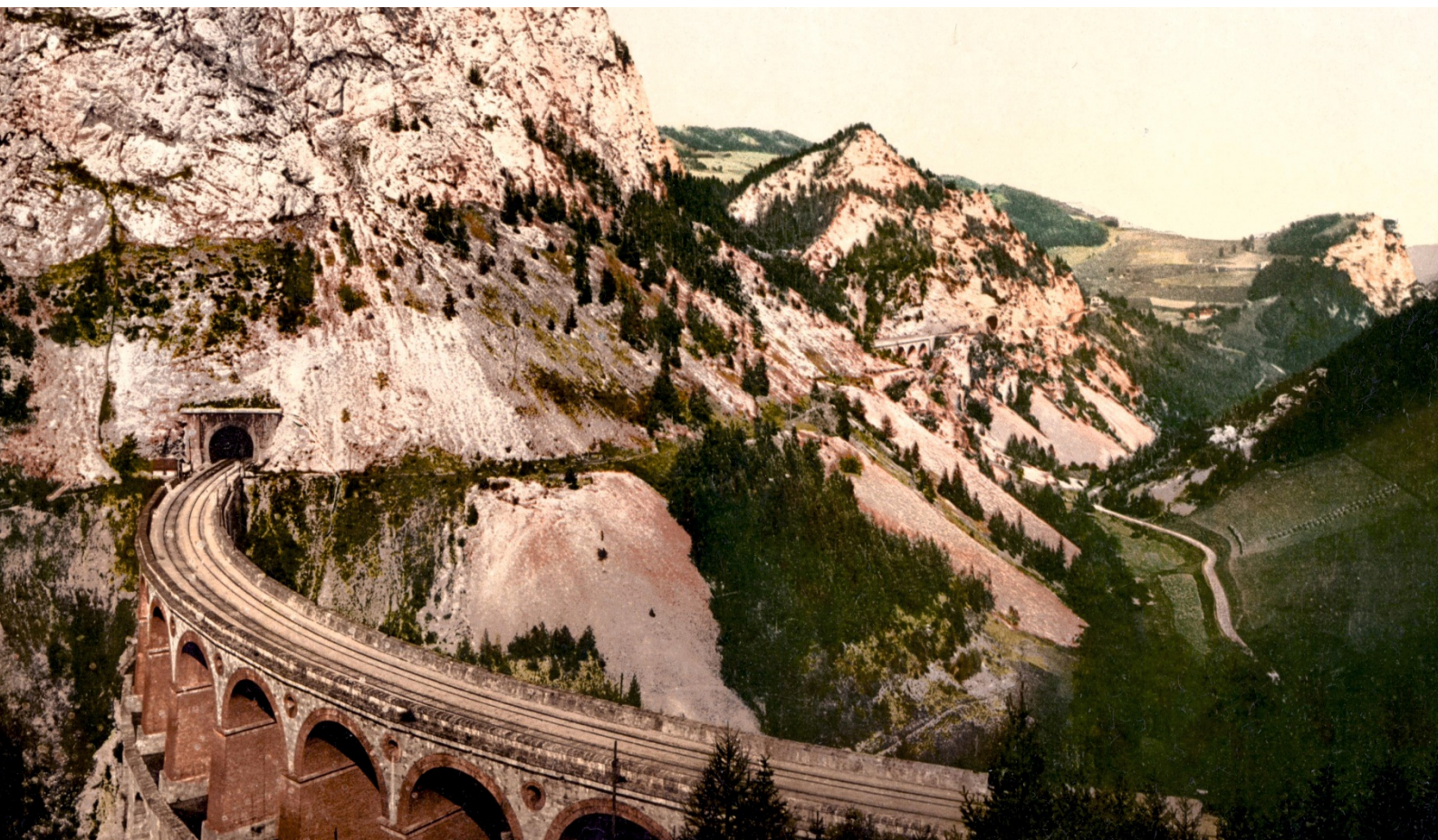
Slika 7. Vijadukt Kalte-Rinne oko 1900. godine (Wikipedia 2019d). Fig. 7. Kalte-Rinne Viaduct, around 1900 (Wikipedia 2019d).
