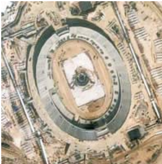
Fig. 1. IKONOS-2 satellite image of Olympic stadium in Athens (URL 2)
